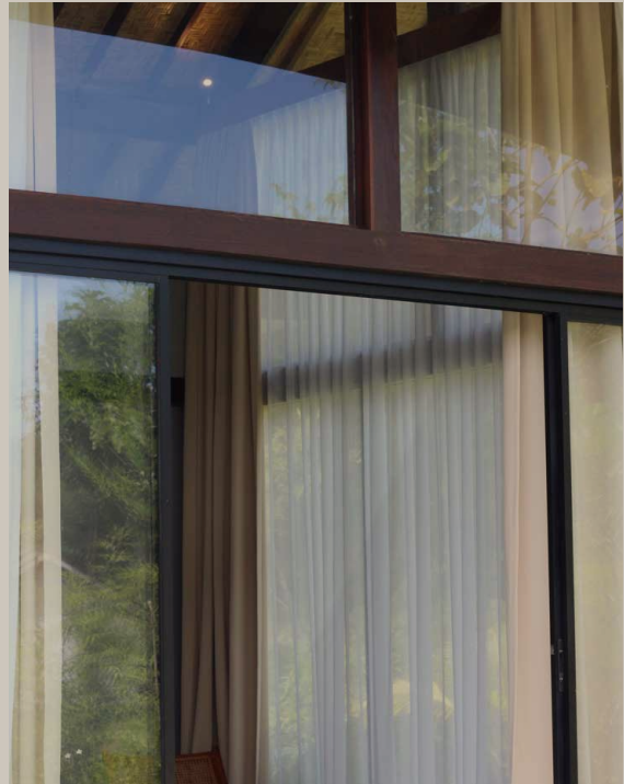
Finishes and detailing reflecting the intended final quality
