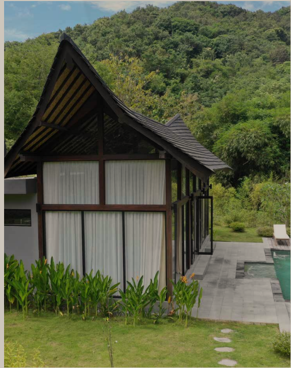
Private villas progressing through active construction
